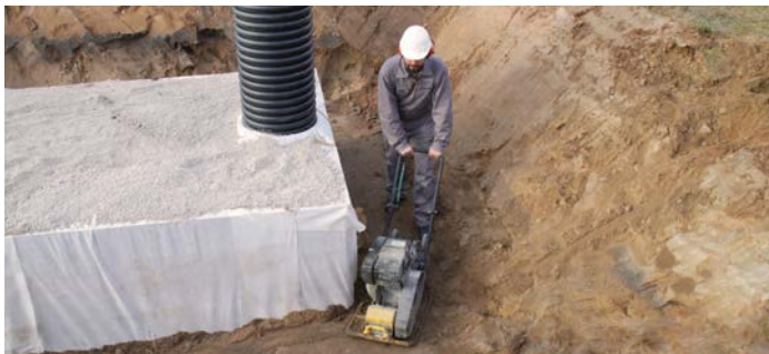
Compression of the working area
