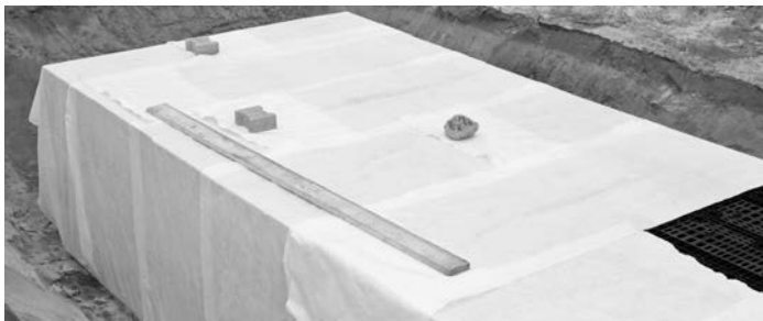
RAUSIKKO Box with geotextile filter
